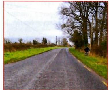
FIGURE 2.3: R163 TO THE NORTHWEST OF ITS JUNCTION WITH THE L74141
