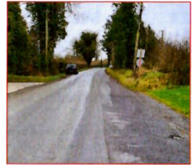
FIGURE 2.2: L74141 IN THE VICINITY OF THE SITE ACCESS
