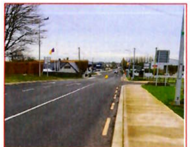
FIGURE 2.4: R162 AT ITS JUNCTION WITH THE R163
